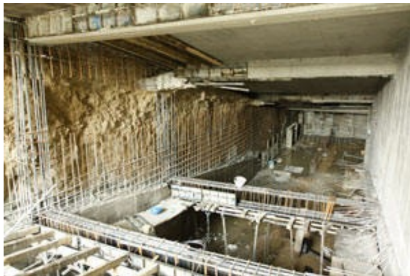
Sahel Sepehr Project - Parking ramp
